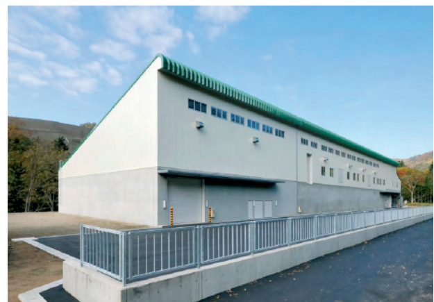
Exterior view of Oshidori Water Treatment Plant Copyright © 2012 JX Nippon Mining and Metals
