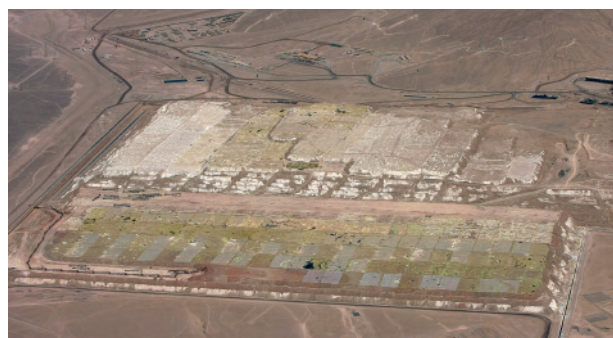
Aerial View of Lomas Bayas leach pads Copyright © 2012 Xstrata
